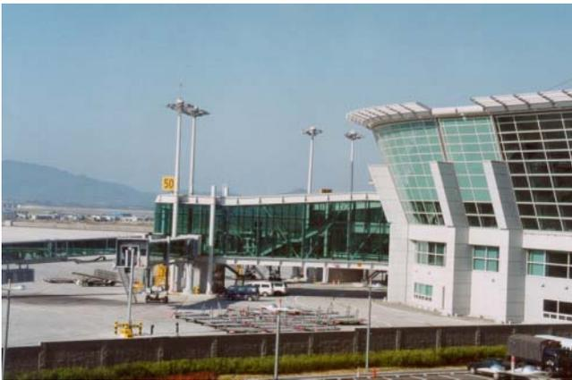
Opened in March 2001, Phase 1 of this state-of-the-art airport offers capacity for 170,000 annual flights, 27 million passengers and 1.7 million tons of cargo using two 3750m close-spaced parallel runways. When fully developed, Incheon International Airport is designed to serve 100 million annual passengers from 4 parallel runways.
